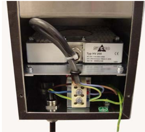
Fig 1. Supply connection terminals
